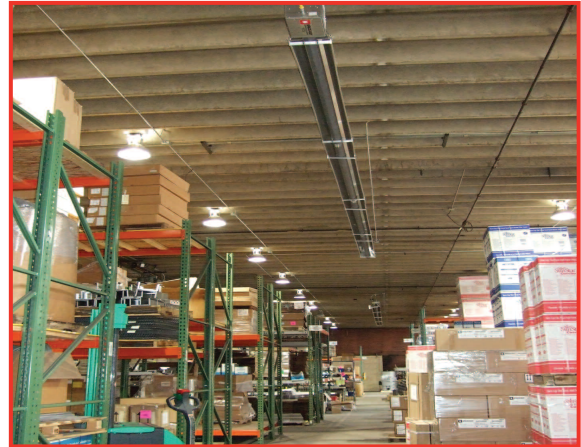
Energy efficient PTS150-40 installed in a manufacturing application.
